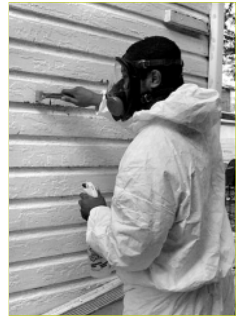
A Healthy Homes inspector performs lead abatement on a Trenton home.
